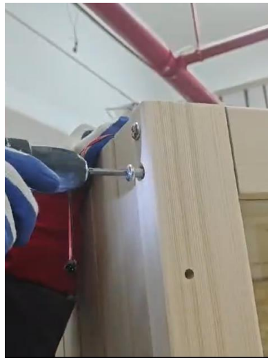
14. Screw the ceiling panel from the side
