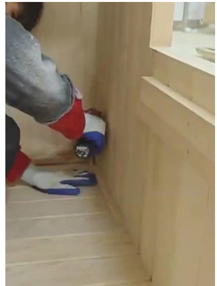
21. Screw the support side when the benches are in place.
