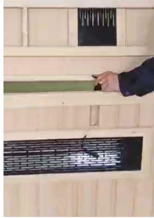
5. Insert the cable for connecting the heaters into the hole at the bottom part of the rear panel.
