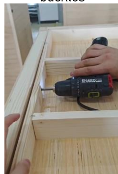
9. Screw the ceiling panel to the upper part of the side panels
