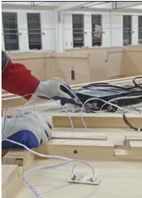
16. Connect the electrical components (see below)
